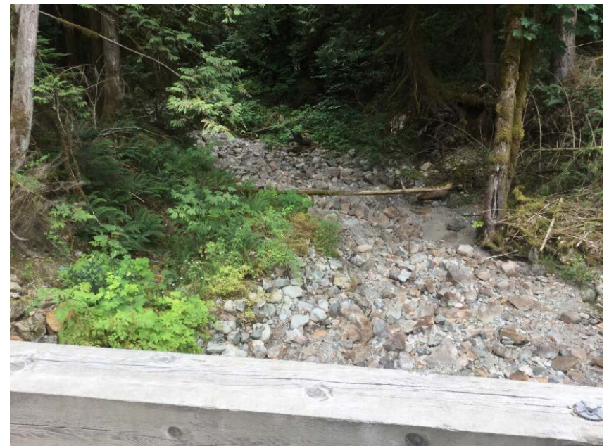
Looking downstream from deck
