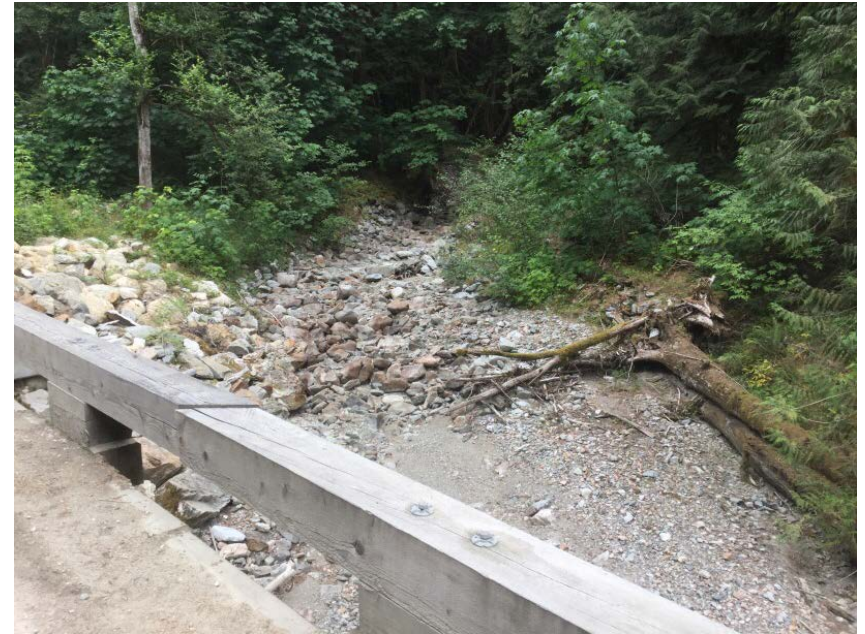
Looking upstream from deck
