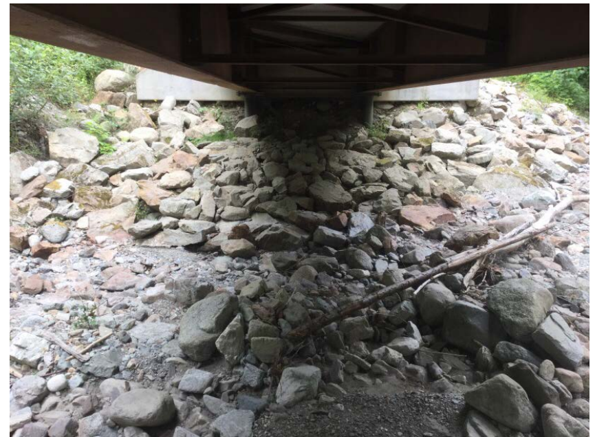
Right Bank Abutment when facing downstream
