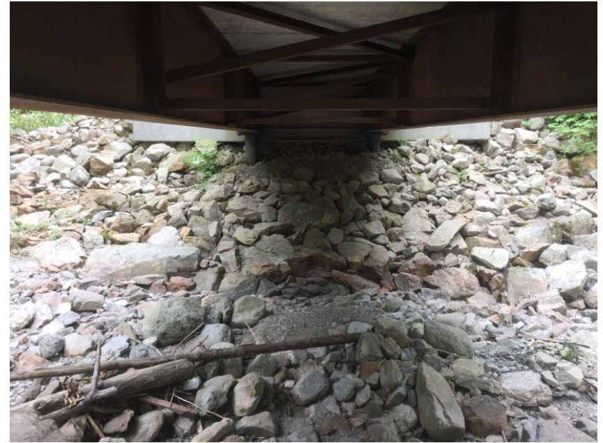
Left Bank Abutment when facing downstream
